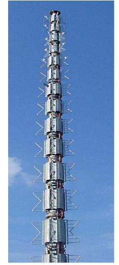
Fig. 1 Horizontally polarized Superturnstile array
