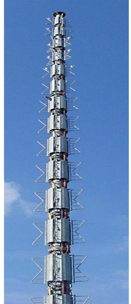
Fig. 1 Horizontally polarized Superturnstile array
