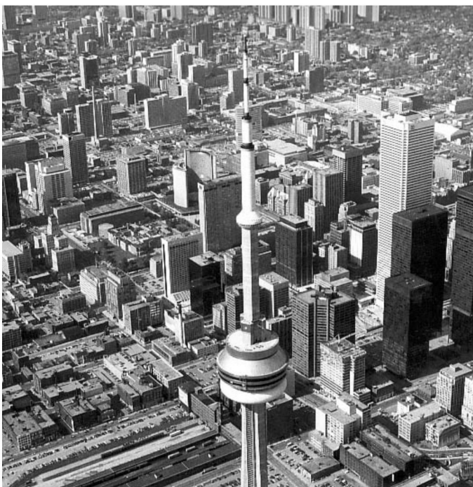
The CN Tower is completed
