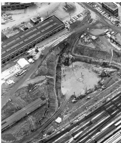
1973, just a hole in the ground
