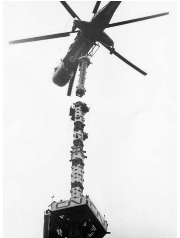
The antenna support spine is lifted into place on the CN Tower
