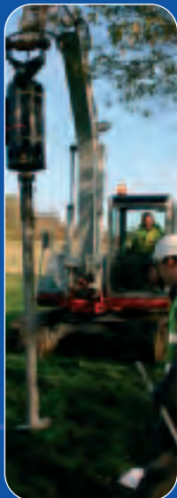
Modular Build – Screwpile
