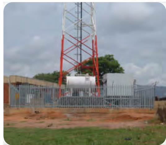
AD9090 TOWER ON QUICKSITE GRILLAGE BASE
