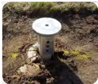
HELICAL PILES ARE DRIVEN INTO GROUND
