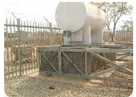
QUICKSITE GRILLAGE BASE: BALLAST 'BASKET' IN POSITION SHOWN WITH NON-INTEGRAL FENCE
