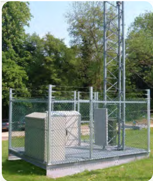
GRILLAGE IS PLACED ONTO PILES, & FENCE, FLOORING, STRUCTURE & CABINETS FITTED (LATTICE TOWER STRUCTURE SHOWN)
