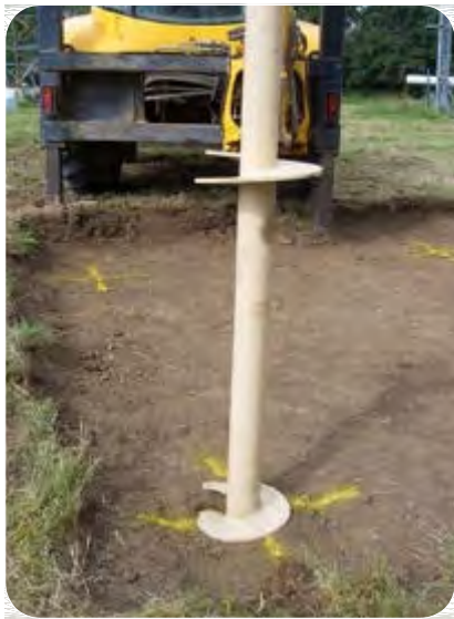
HELICAL PILES ARE DRIVEN INTO GROUND
